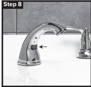
Test the system by passing your hand under the spout (in front of the sensor window) three or four times. The system should prime within 10 activations. If no sound comes from the Pump Pod™, check that all cables and hoses are firmly connected.
