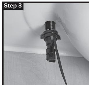
From underneath the counter, feed the lock washer or brass washer and then the mounting nut over the data cable and onto the threaded stem of the dispenser spout. Be sure that the washer will touch the bottom of the countertop and that the nut threads easily onto the stem. (If the nut is hard to turn by hand, it is upside down.) Tighten the nut securely.
