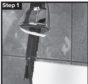
**CX10-P spout:** Remove the paper liner from the bottom of the adhesive gasket to expose the adhesive.
