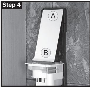
Attach the back plate by first (A) pressing on the top 2 corners and then (B) on bottom middle section. Audible clicks will confirm proper installation.
