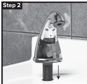
Feed the data cable and the stem of the dispenser spout through the hole in the countertop. Point the spout of the dispenser into the sink bowl. CX10-M spout, skip to Step 3. CX10-P spout, press down firmly on the dispenser spout to securely attach it to the countertop.
