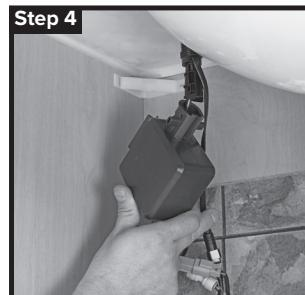
Feed the tube of the Pump Pod™ through the bottom of the stem. Align the indent of the stem to the indent of the Pump Pod™ until it is firmly seated over the base of the stem.
